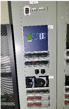
14) Open Air Insulated Station DIFF Relay Bottom Bus Panel
