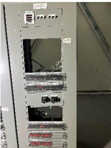
14) Open Air Insulated Station DIFF Relay Bottom Bus Panel
