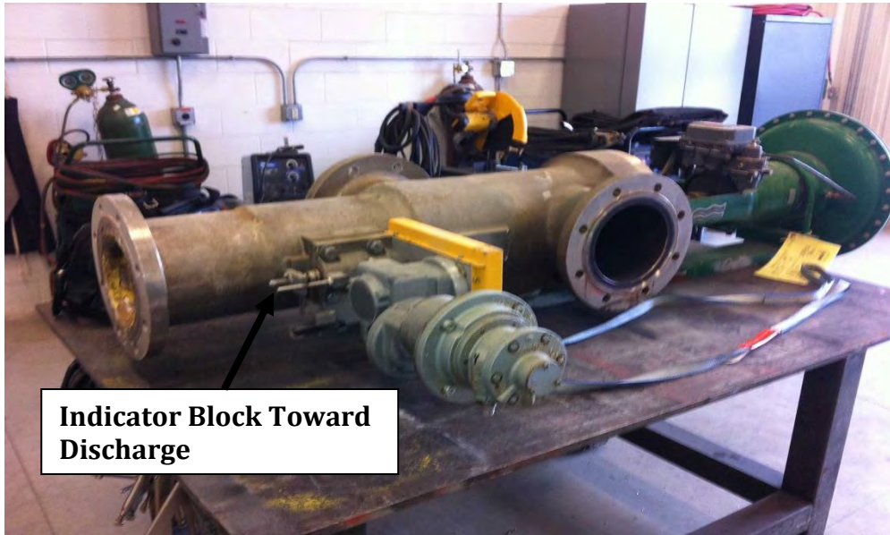
Figure 24: For some older bodies, CTA must be mounted in this direction
